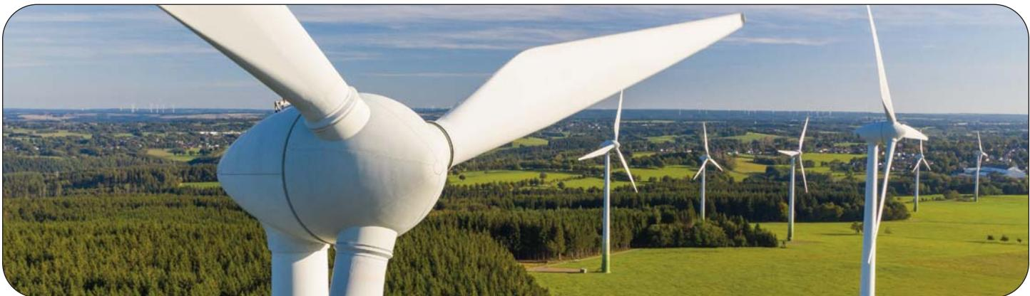
Wind is a domestic source of energy with an abundant and inexhaustible supply. Wind energy has been harnessed for centuries to propel sailing vessels and turn grist mills and water pumps. Today, wind is used increasingly to generate electricity. A wind turbine turns wind energy into electricity using the aerodynamic force from the rotor blades, which work like an airplane wing or helicopter rotor blade.
