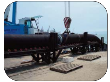
Sand & Gravel Dredging
