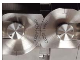
Valve Handle Locking System
