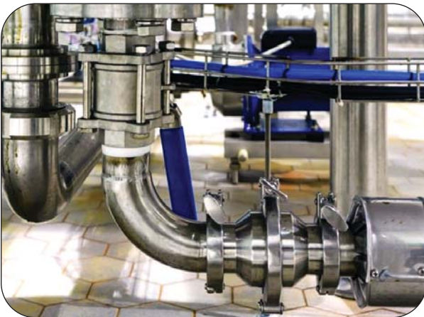
Sanitary flange clamp fitting installed
